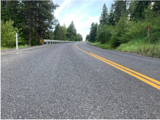
Site 4 (Thorp Prairie Road): Stopping Sight Distance Northbound Vehicle (1500'+ available SSD)
