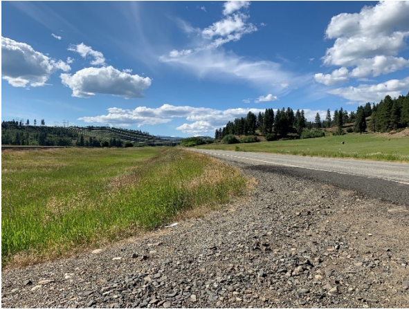
Site 1 (SR 10): Intersection Sight Distance Looking North (1500'+ available ISD)
