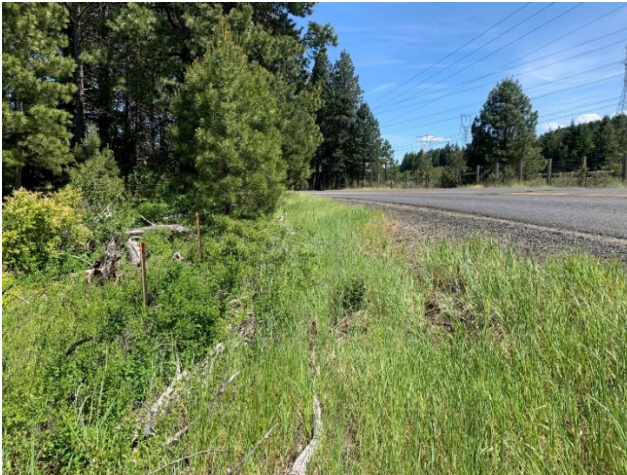
Site 2 (Thorpe Prairie Road): Intersection Sight Distance Looking East (255' available ISD)
