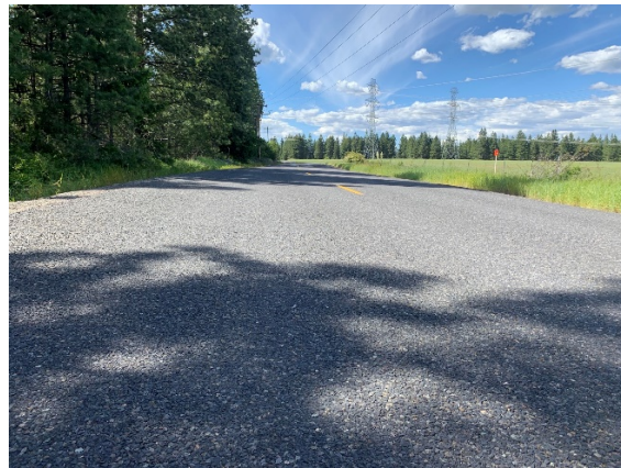
Site 3 (Thorp Prairie Road): Stopping Sight Distance Northbound Vehicle (1000'+ available SSD)
