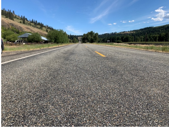
Site 1 (SR 10): Stopping Sight Distance Northbound Vehicle (1500'+ available SSD)
