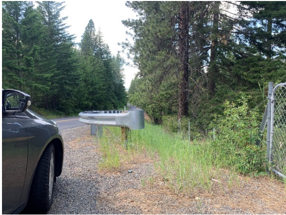
Site 4 (Thorp Prairie Road): Intersection Sight Distance Looking North (625' available ISD)
