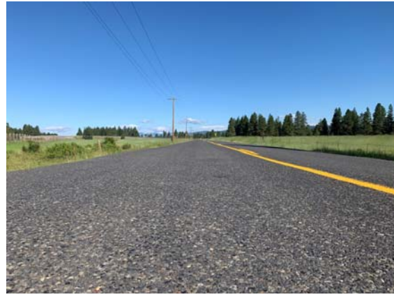
Site 2 (Thorp Prairie Road): Stopping Sight Distance Northbound Vehicle (1000'+ available SSD)
