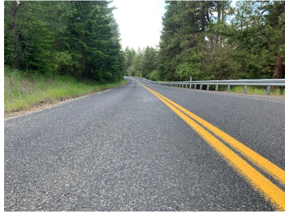
Site 4 (Thorp Prairie Road): Stopping Sight Distance Northbound Vehicle (555'+ available SSD)
