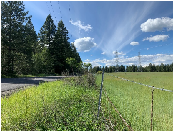
Site 3 (Thorpe Prairie Road): Intersection Sight Distance Looking North (1000'+ available ISD)
