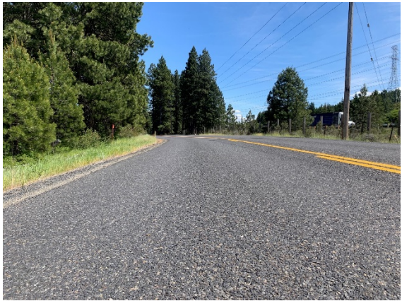
Site 2 (Thorp Prairie Road): Stopping Sight Distance Westbound Vehicle (315' available SSD)
