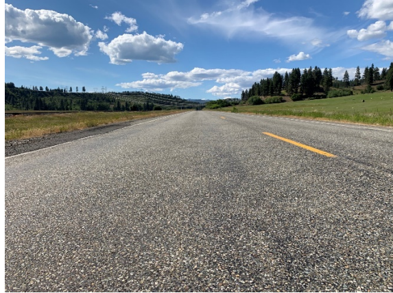
Site 2 (SR 10): Stopping Sight Distance Southbound Vehicle (1500'+ available SSD)
