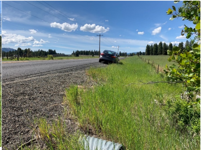
Site 2 (Thorpe Prairie Road): Intersection Sight Distance Looking West (1000'+ available ISD)
