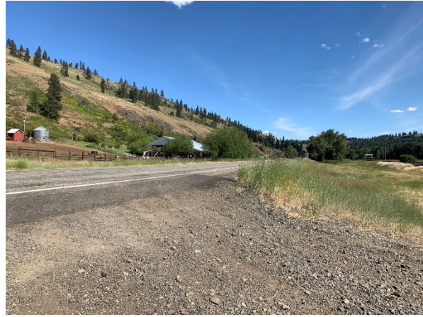
Site 1 (SR 10): Intersection Sight Distance Looking South (1000'+ available ISD)
